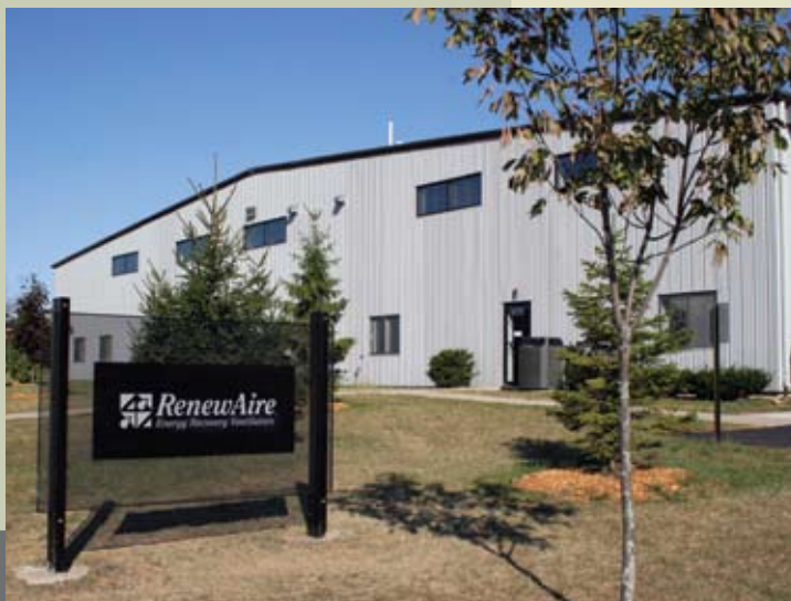
RenewAire offices and manufacturing facility in Madison, WI.
